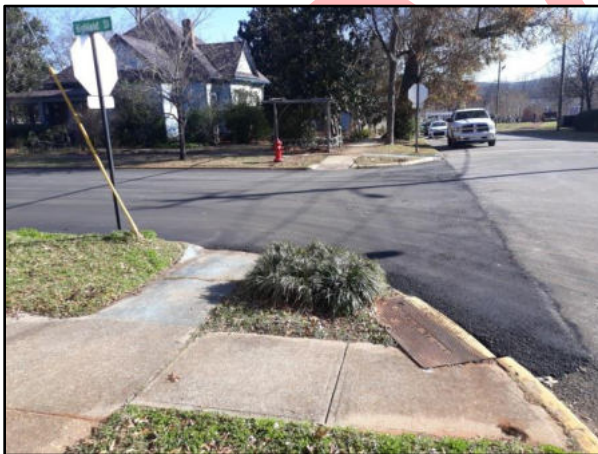
Fig. 8 – 1 older ramp and 1 needed on Bloch St
