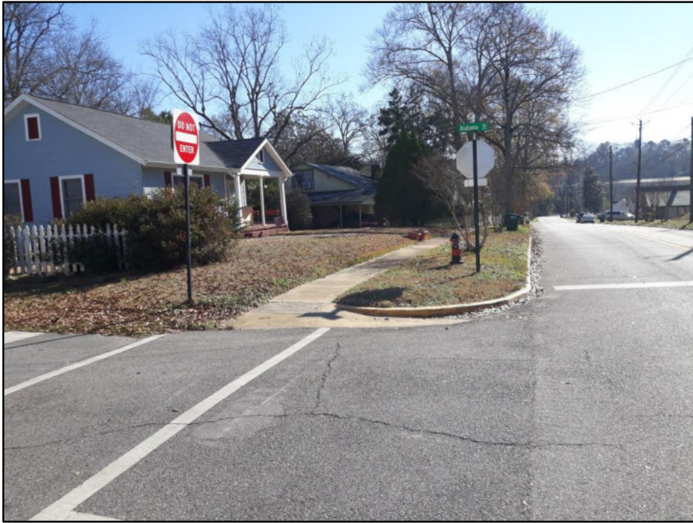
3 – Shelby St at NE corner of Alabama Has updated curb ramp
