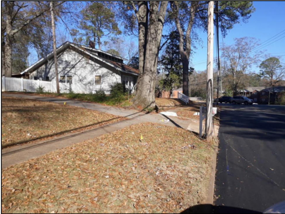
69 – Highland St from Moody to Main Sidewalk cross slope exceeds 2% at one driveway
