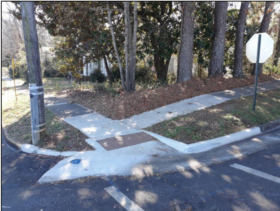
7 – Middle St at Island Updated curb ramps and sidewalk tie ins
