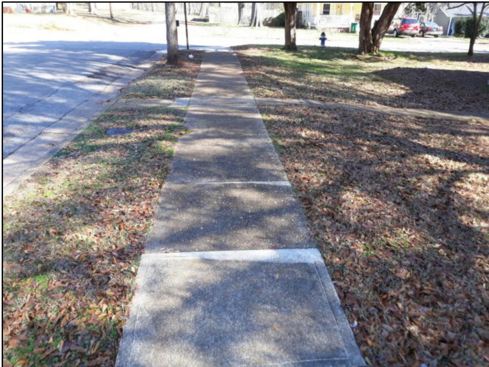
11 – Morgan St from Middle to Vine Sidewalk width =46", has had grinding at panel edges to remove discontinuity
