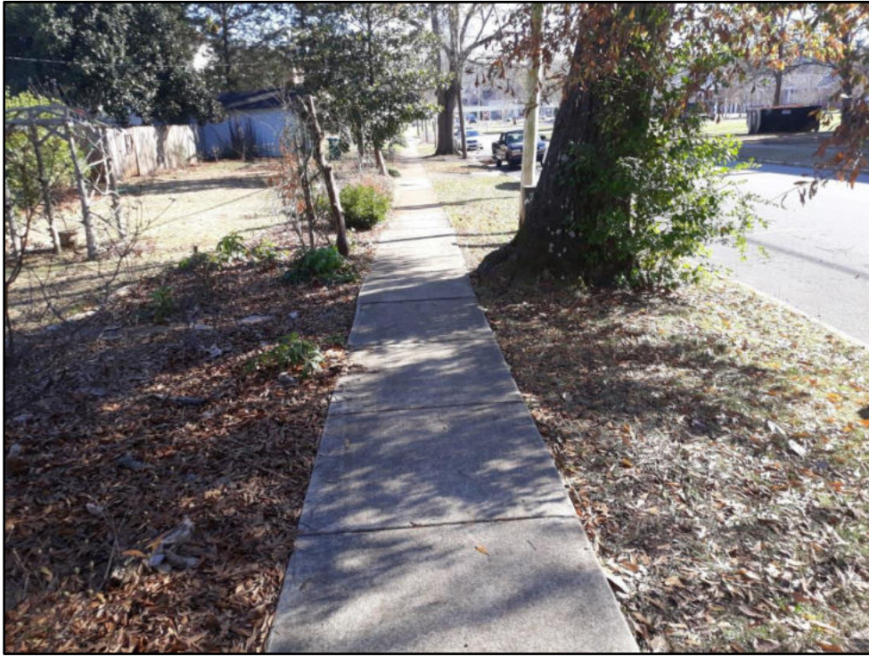
75 – Bloch St from Highland to Oak St Existing sidewalk width is 45”
