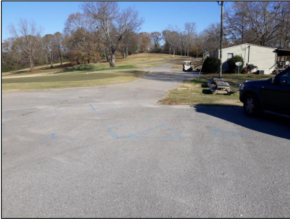
C – Golf Course Has faded ADA parking without signs, no other ADA facilities
