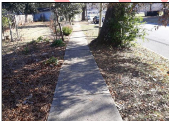
Fig. 4 – 45" width on Bloch St
