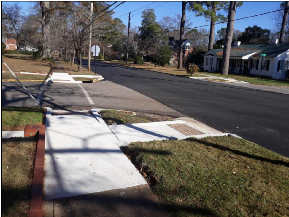
68 – Moody St at Highlands Updated curb ramps and sidewalk tie ins
