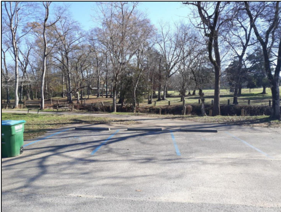
G – Orr Park 3 ADA parking spaces but none that are van accessible with side aisle, parking is not signed
