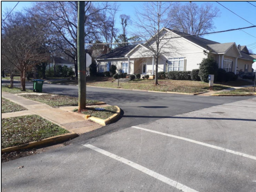
64 – Plowman St at Highland Older sidewalks but does have recently upgraded curb ramps
