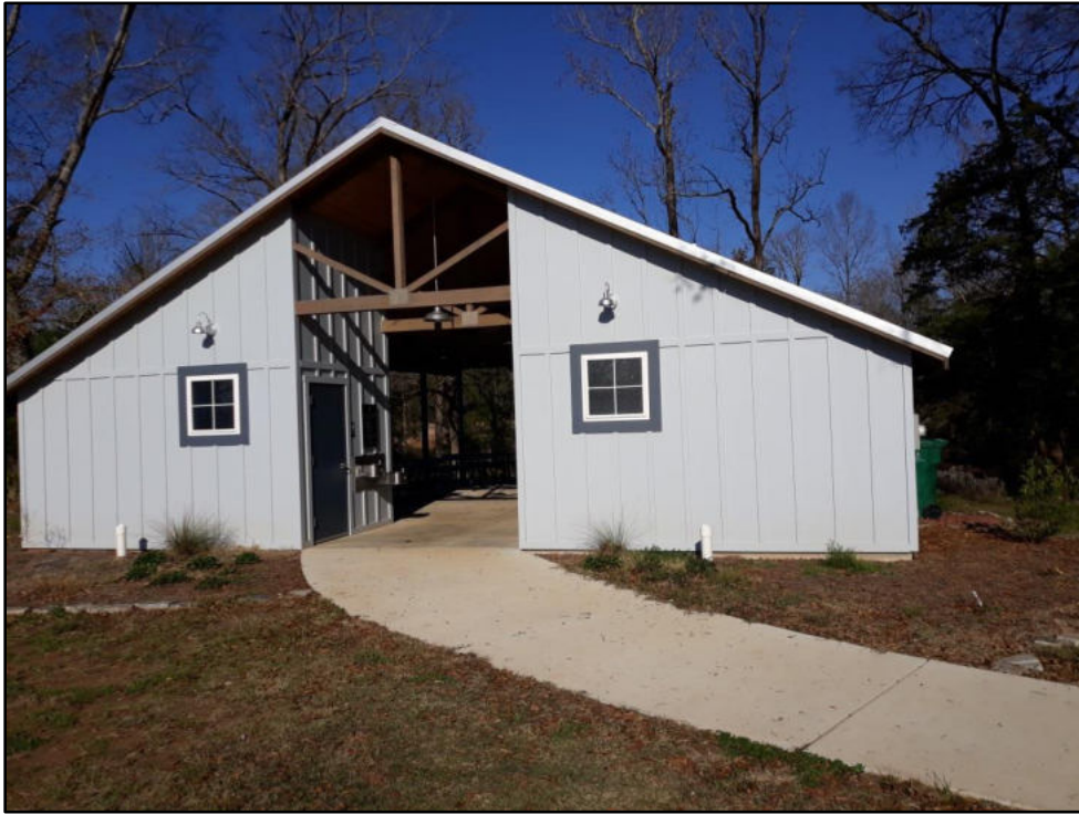
B – Shoal Creek Park Pavillion
