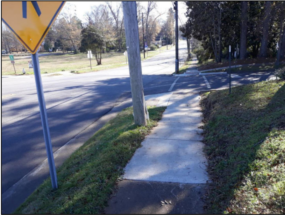
6 – Middle St from Main to Island Existing sidewalk width is 44”
