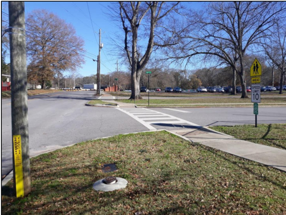
14 – Island St at Park Good sidewalk and cross walk with updated curb ramps
