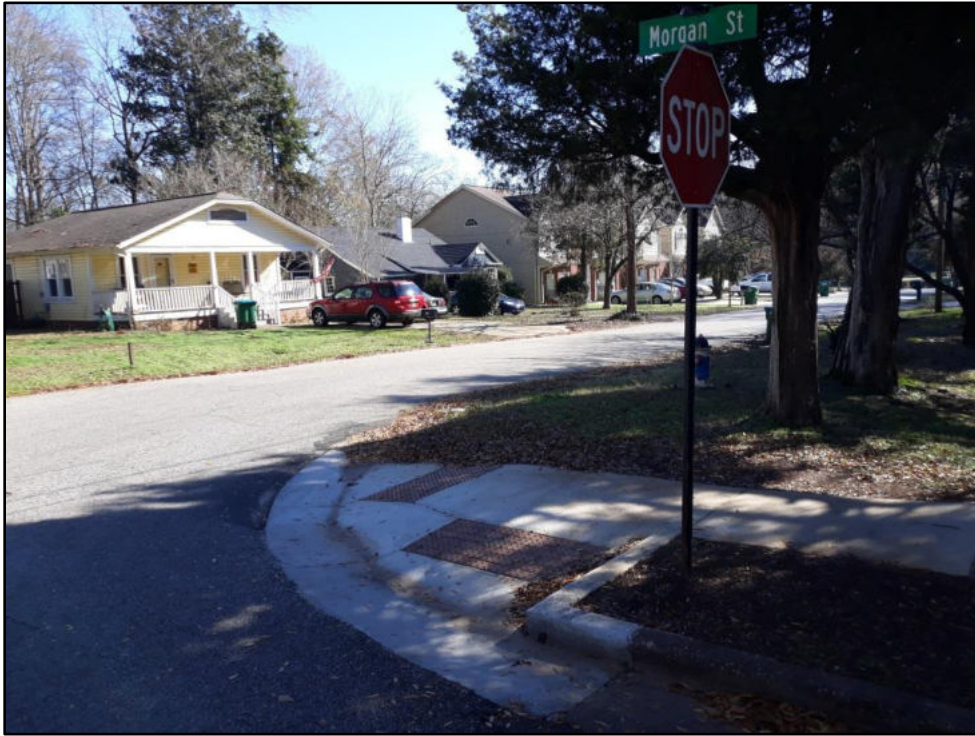
12 – Morgan St at Vine Updated curb ramps and sidewalk tie ins
