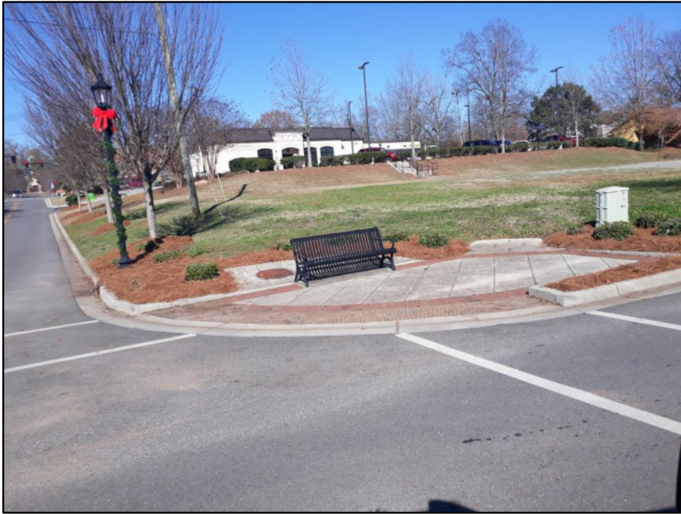
13 – Island St at N Boundary Good sidewalk and cross walks with updated curb ramps
