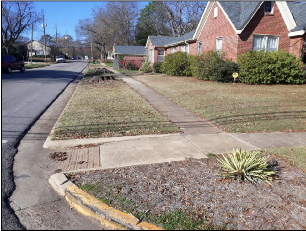
64 – Plowman St from Oak to Highland Older sidewalks that are 48", utilize driveway as a passing zone, have had updated curb ramps
