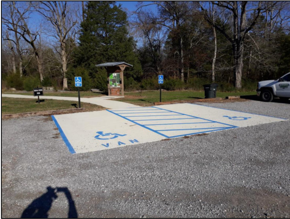
B – ADA parking spaces at Shoal Creek Park Good level areas, well Stiped & signed, good access aisle
