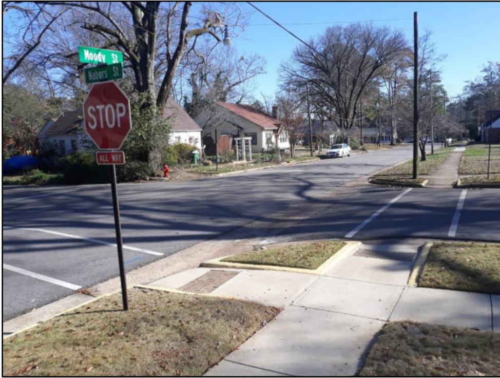
67 – Moody St at Nabors Has updated curb ramps and some replaced sidewalk panels
