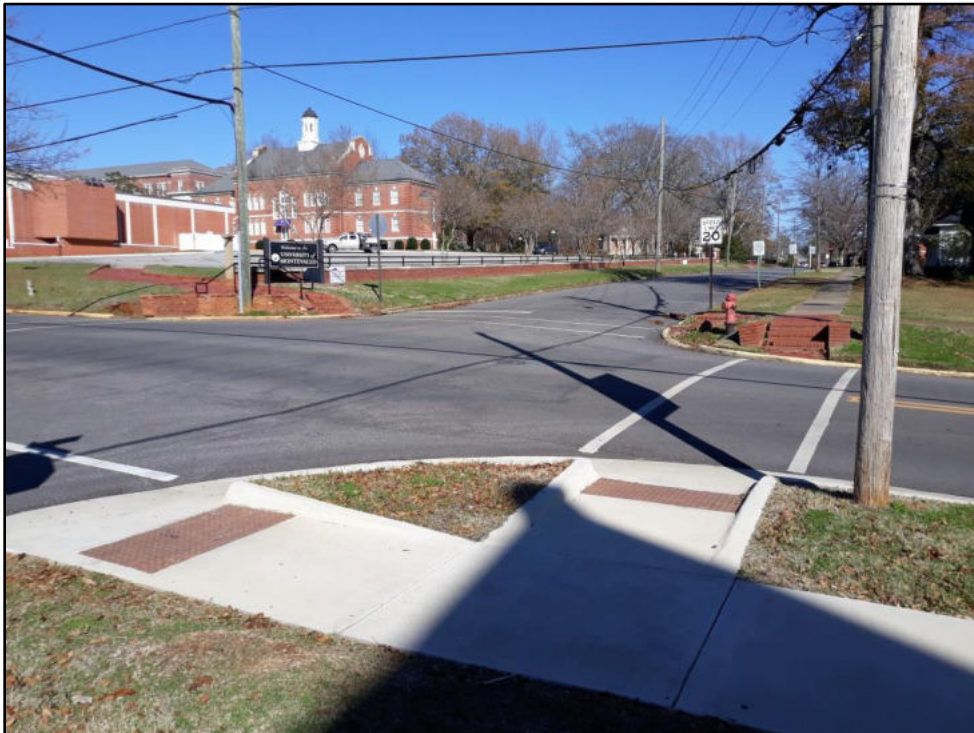
52 – Middle St at Oak Updated ADA ramps and sidewalk tie ins, steps across Middle are owned by University
