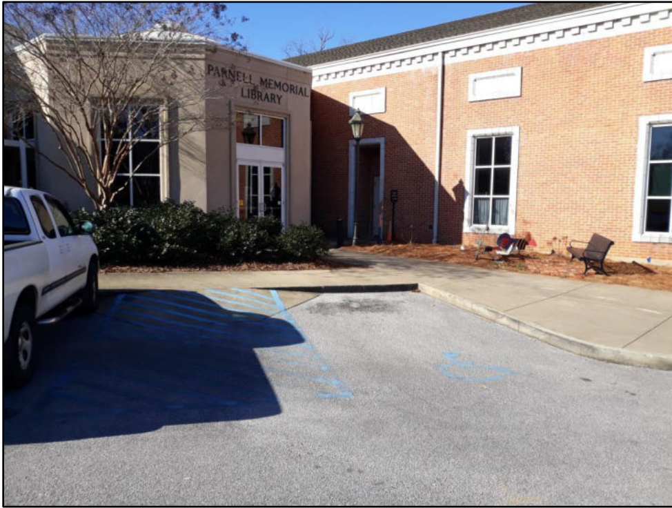
F – Library Has 2 ADA parking spaces, parking is not signed
