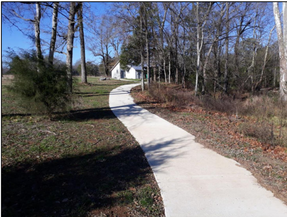
B – Pedestrian route from parking to pavilion at Shoal Creek Park Good width and cross slope
