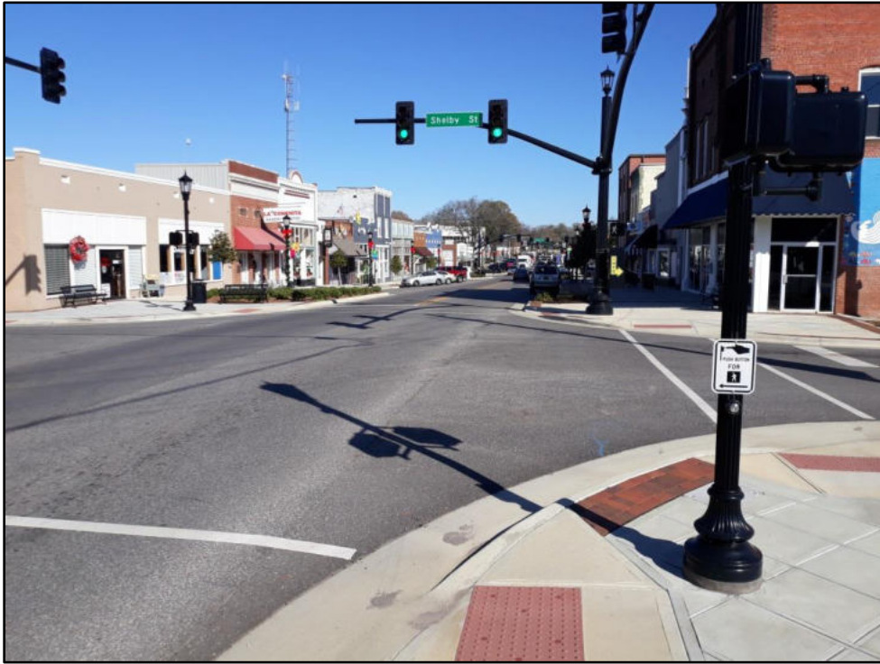
21 – Main St at Shelby Good recent construction of sidewalk, ramps, cross walks, and pedestrian signals
