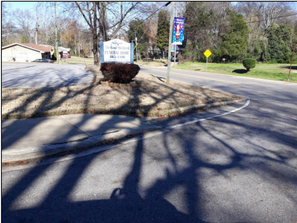
19 – White St at Hwy 119 Ramp needs to be updated to current standards
