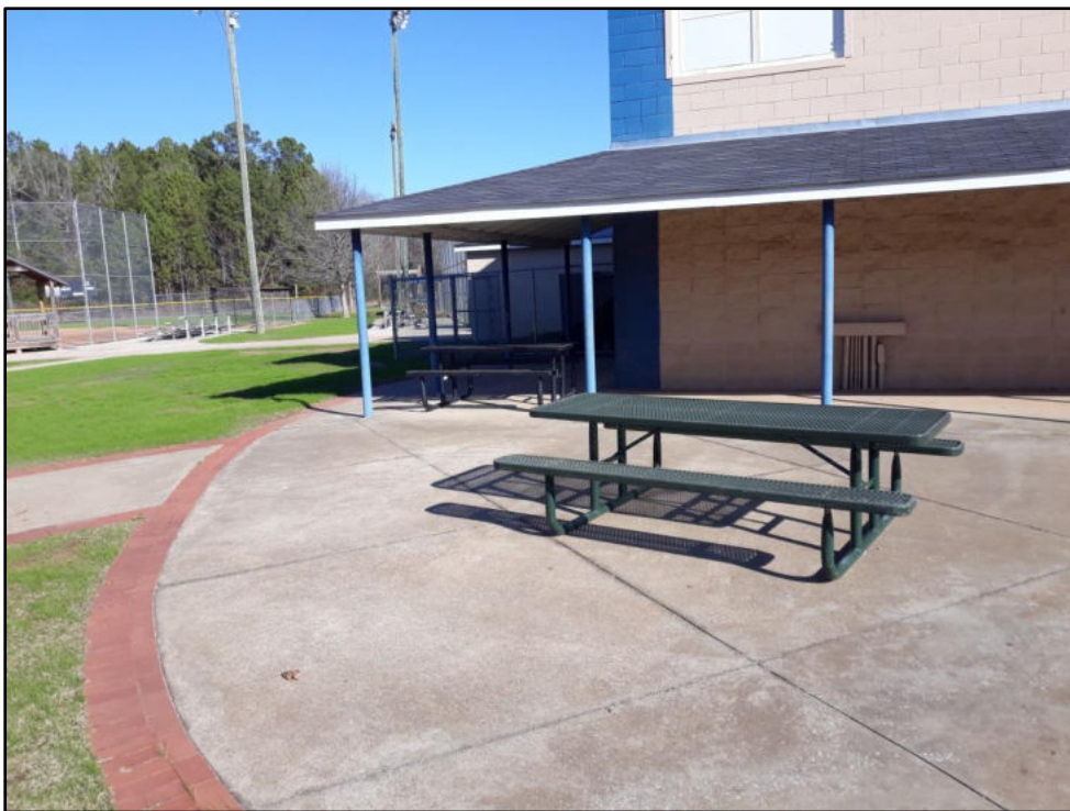
D – Stephens Park Good ADA compliance, 2 picnic tables with extended ends for wheelchair access
