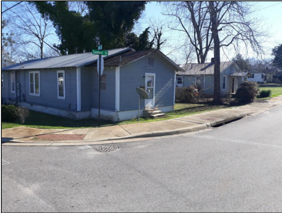
18 – White St at Samford Recent curb ramps but without a level turning space so cross slope exceeds 2%
